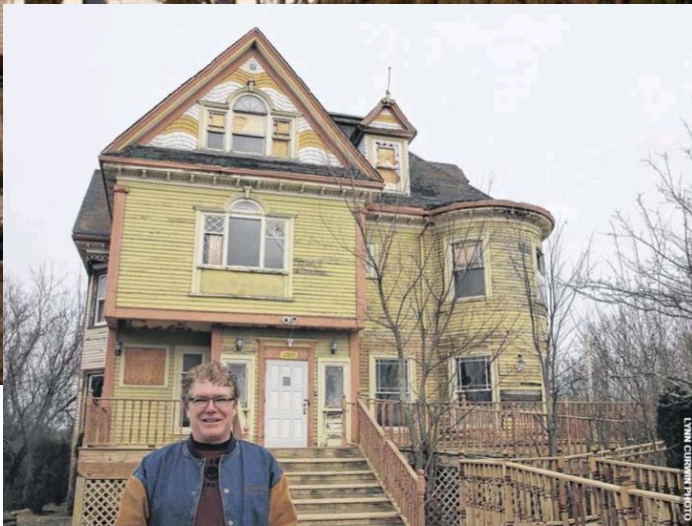
Paul Blenkhorn has been busy working on the former John Stanfield Inn. He bought the building this fall and plans to live in it, as well as offer rooms and apartments for rent, once restoration is complete.
